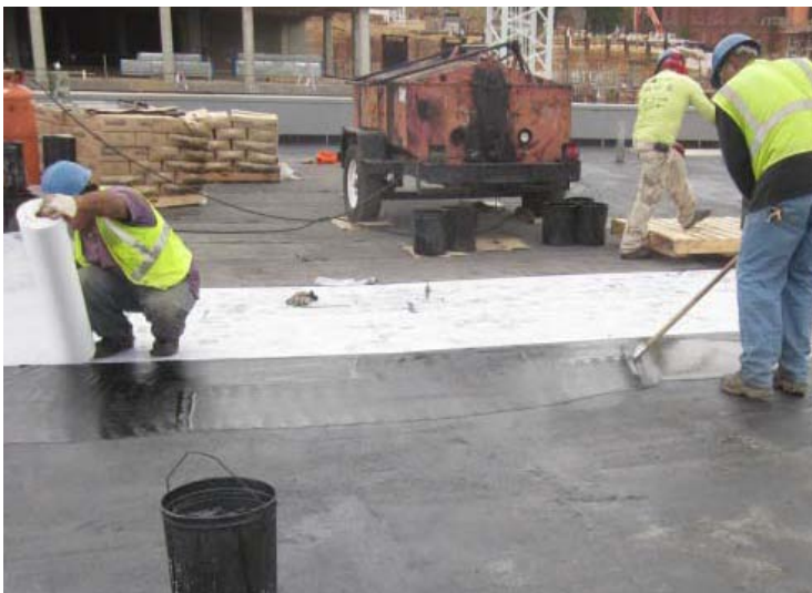
Crews installing hot rubberized asphalt.
