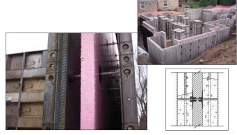
Thermomass System CIP, vertical cast, with FOAMULAR® Insulation
