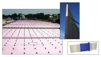
Thermomass System SC, tilt-up with FOAMULAR® 250
