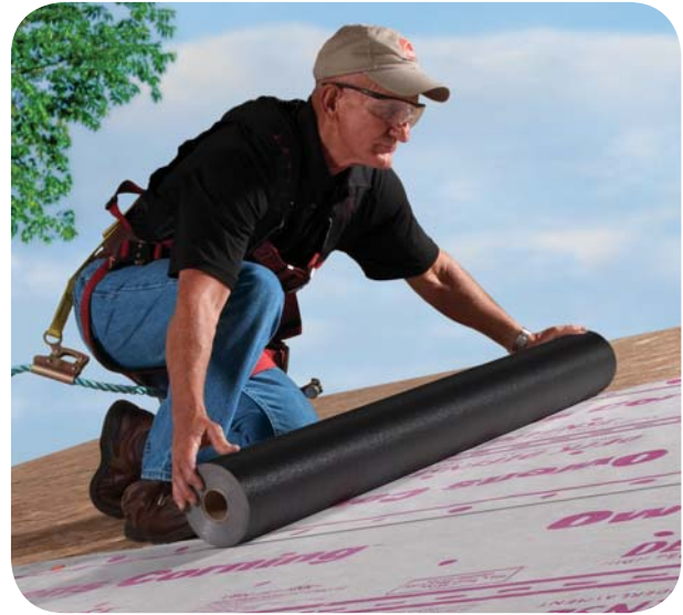
Figure 1: Typical Underlayment Installation
