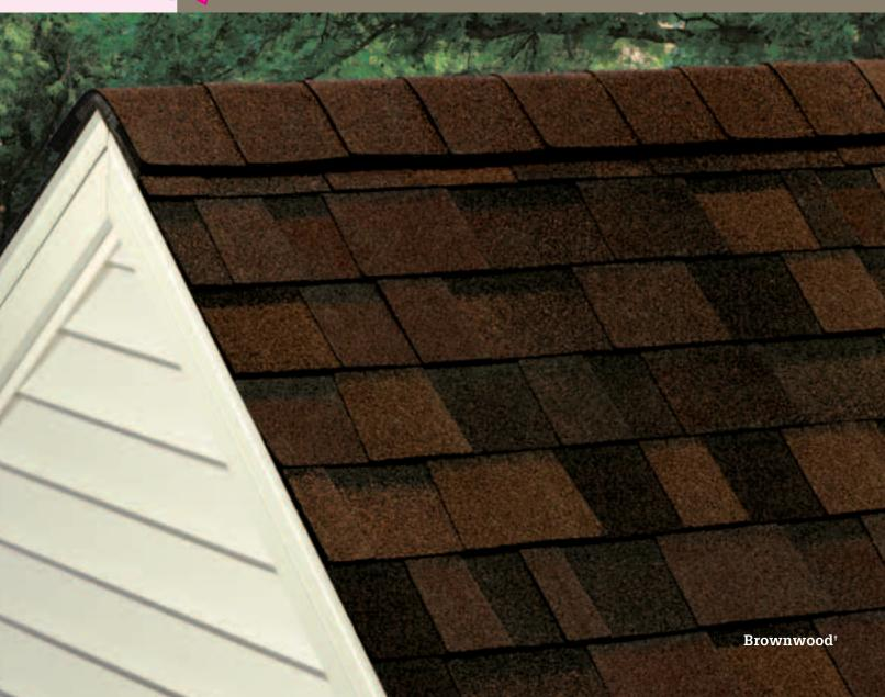
Owens Corning™ Perforated Hip & Ridge Shingles with Sealant add excellent protection and long-lasting beauty to your roof's peak. It also comes in perforated "tabs," making your job faster and simpler.
