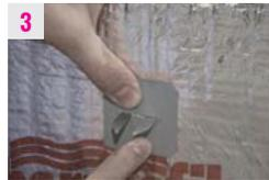
3 A locking washer is slid over the hanger to fit tightly against the insulation panel.
