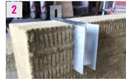
2 The forked leg of the hanger provides a shelf-like ledge to support the insulation.
