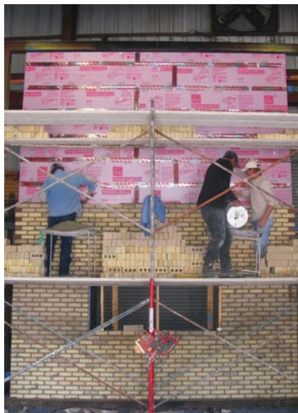
NFPA 285 test wall under construction.
