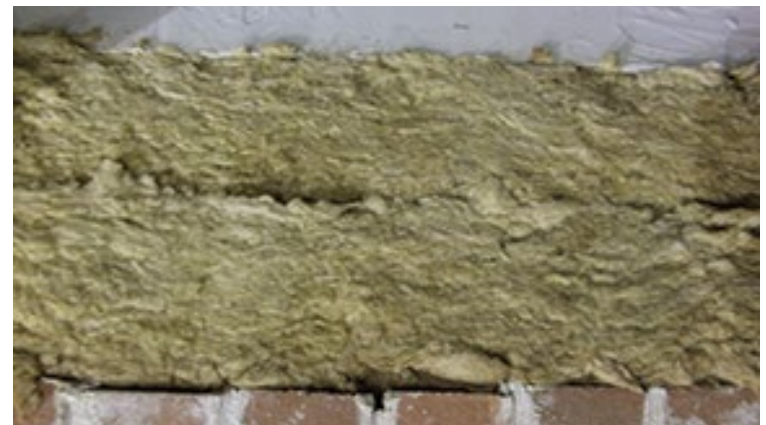
Thermafiber® Safing is compression fitted between exterior masonry and the exterior gypsum sheathing, or, the concrete slab edge to create a perimeter fire containment system.
