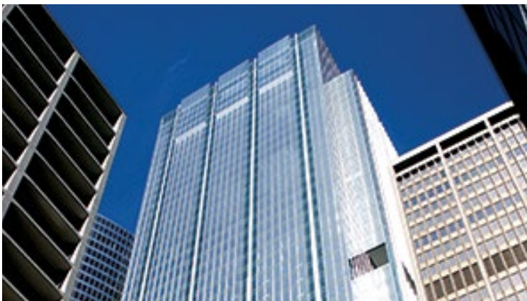
Thermafiber® Safing and FireSpan® insulation provide the critical components of the perimeter fire containment system in the 111 South Wacker Building in Chicago, IL. Thermafiber insulation also contributed to the building's LEED® Gold Rating.
