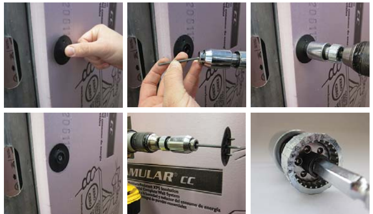
Prevents screw wobble Depth adjustment dial
