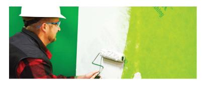
Other components of the CavityComplete® Wall System, Owens Corning® FOAMULAR® Extruded Polystyrene (XPS) Insulation, Mortar Net Solutions™ TotalFlash® and/or Tremco® accessory materials may be installed after the ExoAir® 230 membrane has fully cured, approximately 16-24 hours, or is firm and dry to touch.
