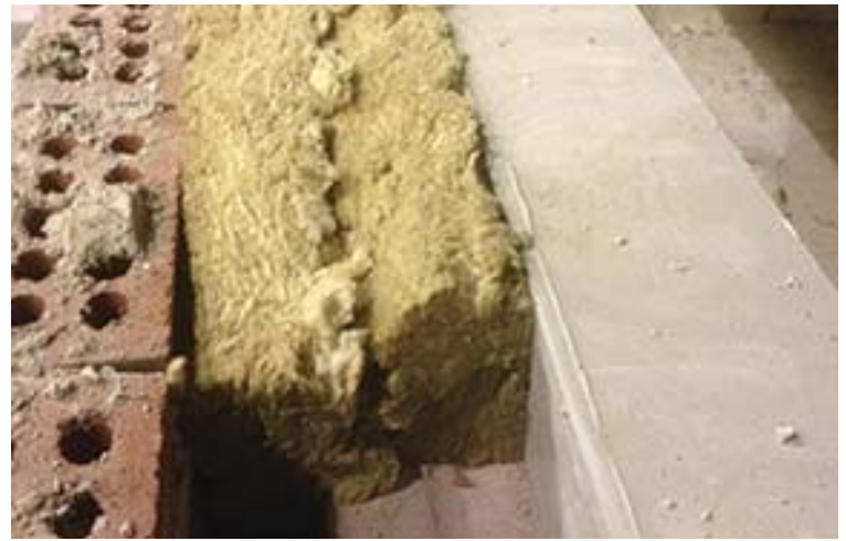
Figure 2: Correct Compression Installation around an opening in a wall with masonry veneer.
