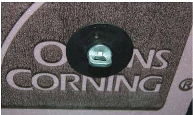
Pos-I-Tie® Barrel screw and Rodenhouse Thermal-Grip® washer
