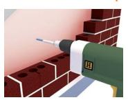
Install the Original Pos-I-Tie® into the backup wall using a chuck adapter and power drill.
