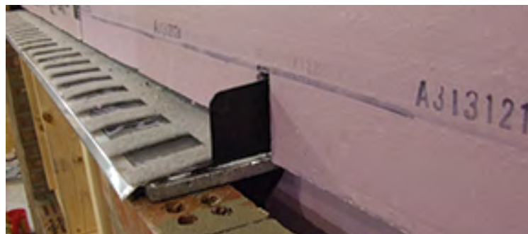
TotalFlash® flashing preassembled unitized through wall flashing/drip edge assembly installed over continuous steel brick ledge.
