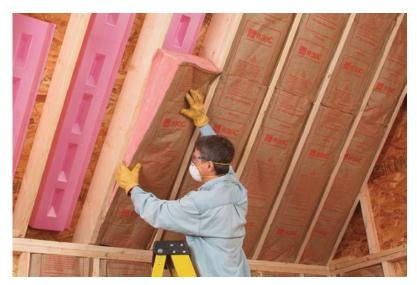
EcoTouch<sup>®</sup> Insulation is easy to handle and install. Sized for installation in either wood or metal frame construction, EcoTouch<sup>®</sup> Kraftfaced Insulation can be friction fit or stapled into place. Trimming and fabrication can be done with an ordinary utility knife and is easily installed into odd-shaped cavities and small spaces. With less dust than other fiberglass insulation products, EcoTouch<sup>®</sup> Insulation has excellent stiffness and recovery characteristics.
