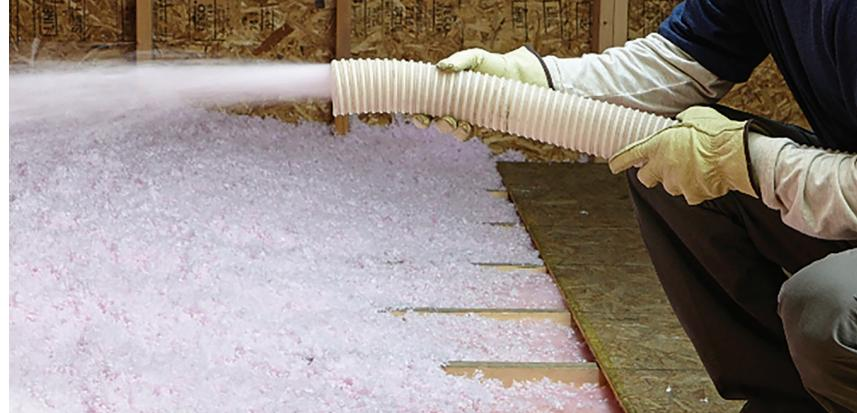
AttiCat® PINK® Blown-In Insulation is a loosefill Fiberglas™ thermal insulation. It is designed for use exclusively with the AttiCat® machine.
