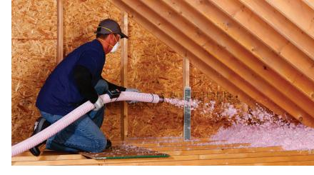
ProCat® Insulation is a loosefill fiberglas™ thermal insulation. It is designed for use exclusively with the ProCat® machine.
