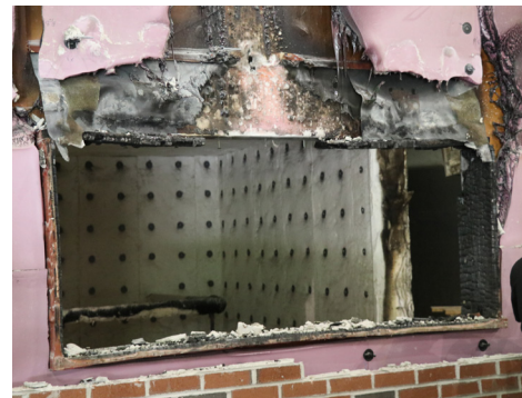
Figure 5: FOAMULAR® NGX® showing limited damage above the test window with brick veneer stripped away after the fire test
