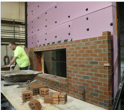
Figure 3: FOAMULAR® NGX® test wall under construction
