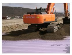
The runway at Thule Air Force Base had experienced damage from permafrost thaw. In 2015, Thule Air Force Base completed a runway rehabilitation project that incorporated Owens Corning® FOAMULAR® GEO 60 psi extruded polystyrene geofoam insulation to prevent damage at the most critical locations, or approximately 18 percent of the runway.
