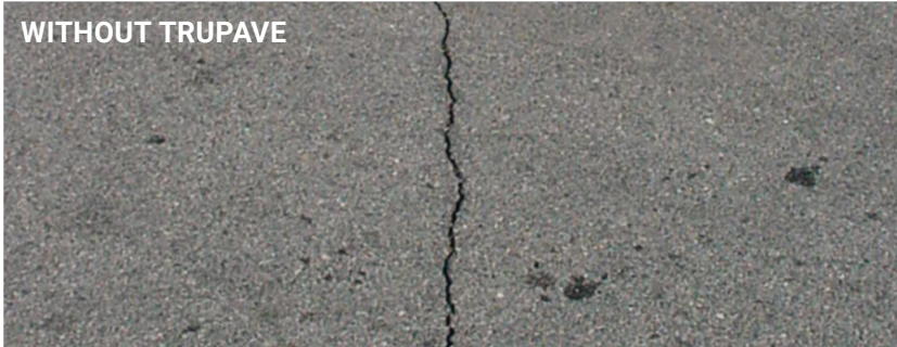
Lakeland, FL: Installed February 2001 Soil Cement Base | Overlay over HMAc | Cracking stops at TruPave
