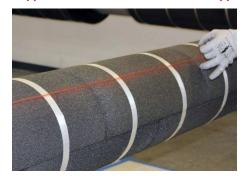
**Step 1**After FOAMGLAS® insulation is installed, strike a horizontal line along the insulation convenient for starting jacket positioning and to ensure a uniform lap line.
