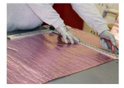
**Step 2**Cut a length of jacketing to provide at least a 2 in. (50 mm) overlap at the longitudinal seam.
