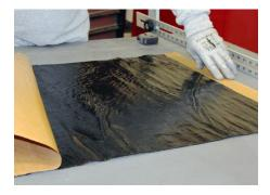
**Step 3**Slit the release film at this overlap, taking care not to slit jacket. Remove release film except at the overlap. Dirt and dust must be kept off jacketing.
