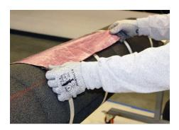
**Step 4**Starting on the chalk line, press the surface of the jacketing halfway around the FOAMGLAS® insulation.
