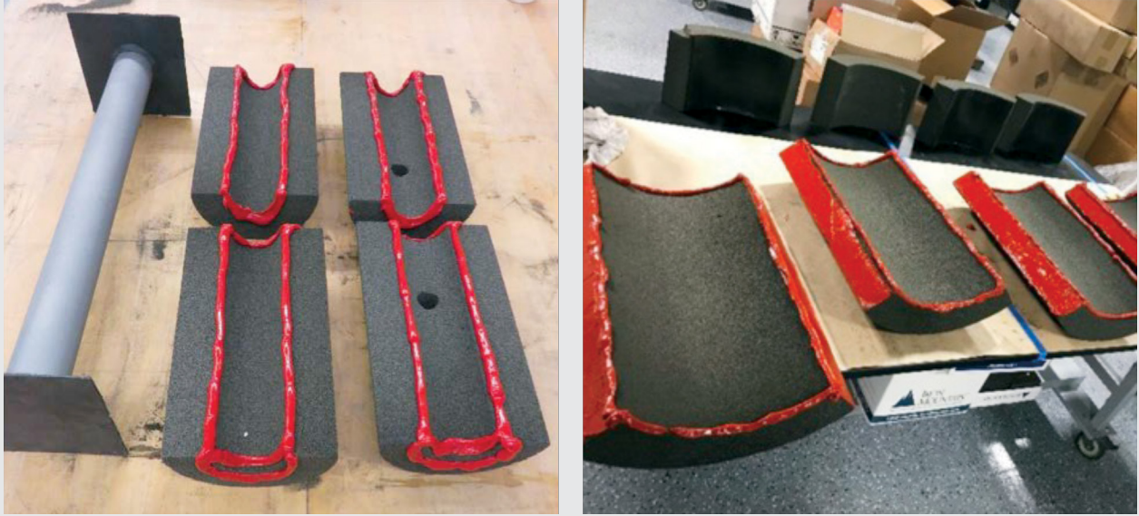
Figure 6 – For the best protection, sealant needs to be correctly applied.
