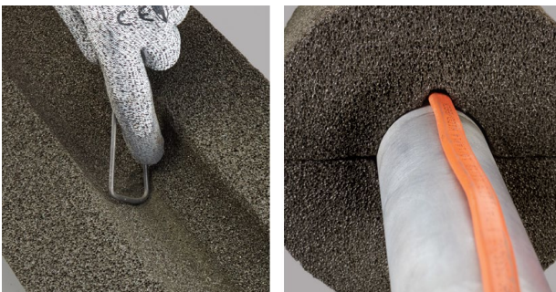
Application over trace heating
