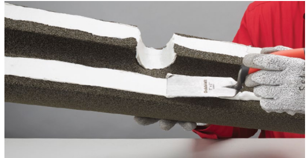
Spreading of joint sealants to full-depth
