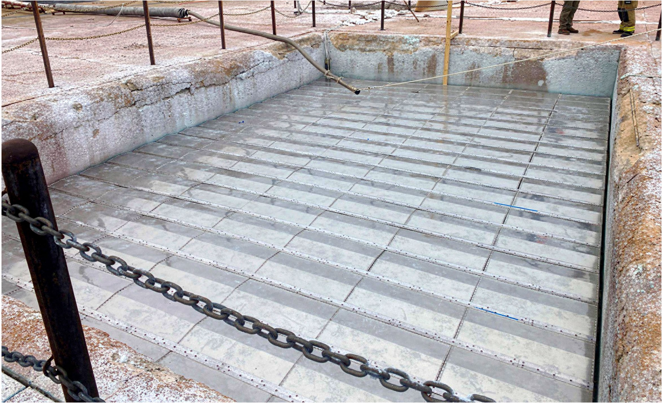
Figure 9. Gen 2 PFS blocks installed in the LNG impoundment.
