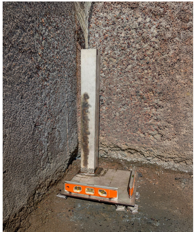
Figure 5. Thermocouple tree: as installed in the impoundment.
