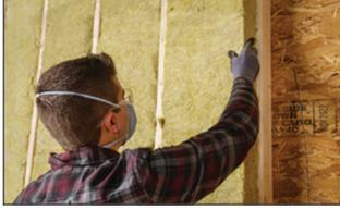
**Thermafiber® Fire & Sound Guard® Plus** mineral wool insulation is designed to provide excellent thermal, noise control, and fire resistance in residential and light commercial construction applications. Fire & Sound Guard® Plus can be used in a variety of applications, including interior and exterior walls, ceilings, basement walls, and crawl spaces. These products are non-combustible, moisture-resistant, non-corrosive, non-deteriorating, and mold-resistant<sup>2</sup>.
