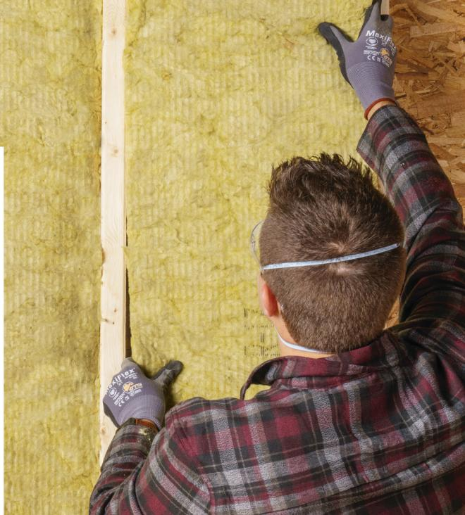
Thermafiber® Fire & Sound Guard® Plus is a hybrid light-density mineral wool batt designed for use in both interior and exterior wall cavities. It offers a combination of thermal and acoustic performance that streamlines installation.
