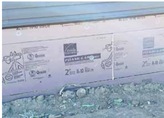
Figure 15: Below-grade exterior insulation showcasing 51 mm (2') FOAMULAR® C-300 Extruded Polystyrene Rigid Insulation. Source: SAIT
