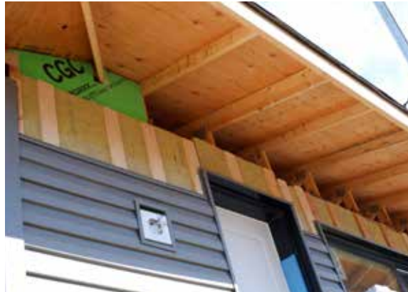
Figure 13: Photo of exterior 51 mm (2') Thermafiber® RainBarrier® ci High Compressive Plus (110) Mineral Wool Insulation and strapping below vinyl cladding. Source: SAIT
