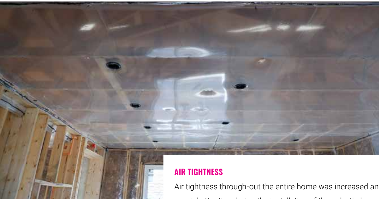
Figure 3: Photo of living room ceiling with pot-lighting taken during blower door test 1. Source: primary
