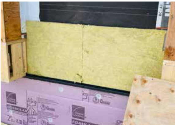
Figure 14: Below-grade to above grade wall transition showcasing 51 mm (2') Thermafiber® RainBarrier® ci High Compressive Plus (110) Mineral Wool Insulation and 51 mm (2') FOAMULAR® C-300 Extruded Polystyrene Rigid Insulation. Source: SAIT
