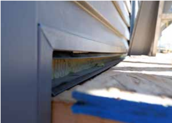
Figure 12: Photo of double flashing and insulation detailing around attached deck at rear of home. Source: SAIT
